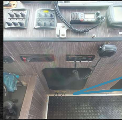
Port and Starboard Fuel Shut Off
